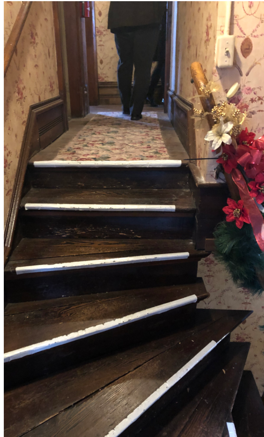
Existing winding stairs at top portion of main stair
